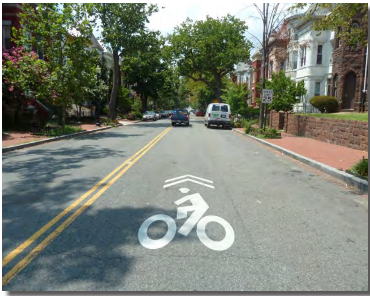
Shared Lane Marking
