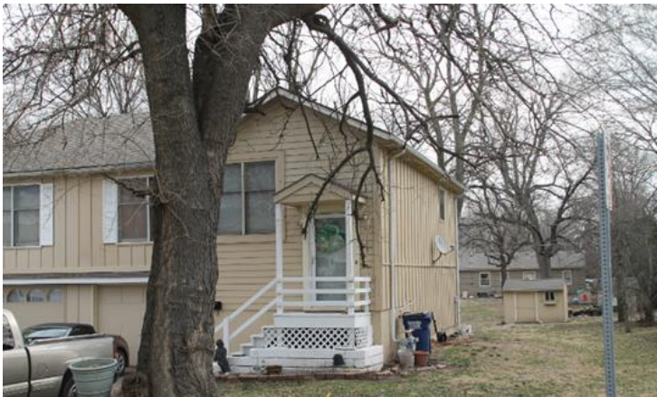
Exhibit 4: Original front porch with a three-foot encroachment (picture from March 2016)
