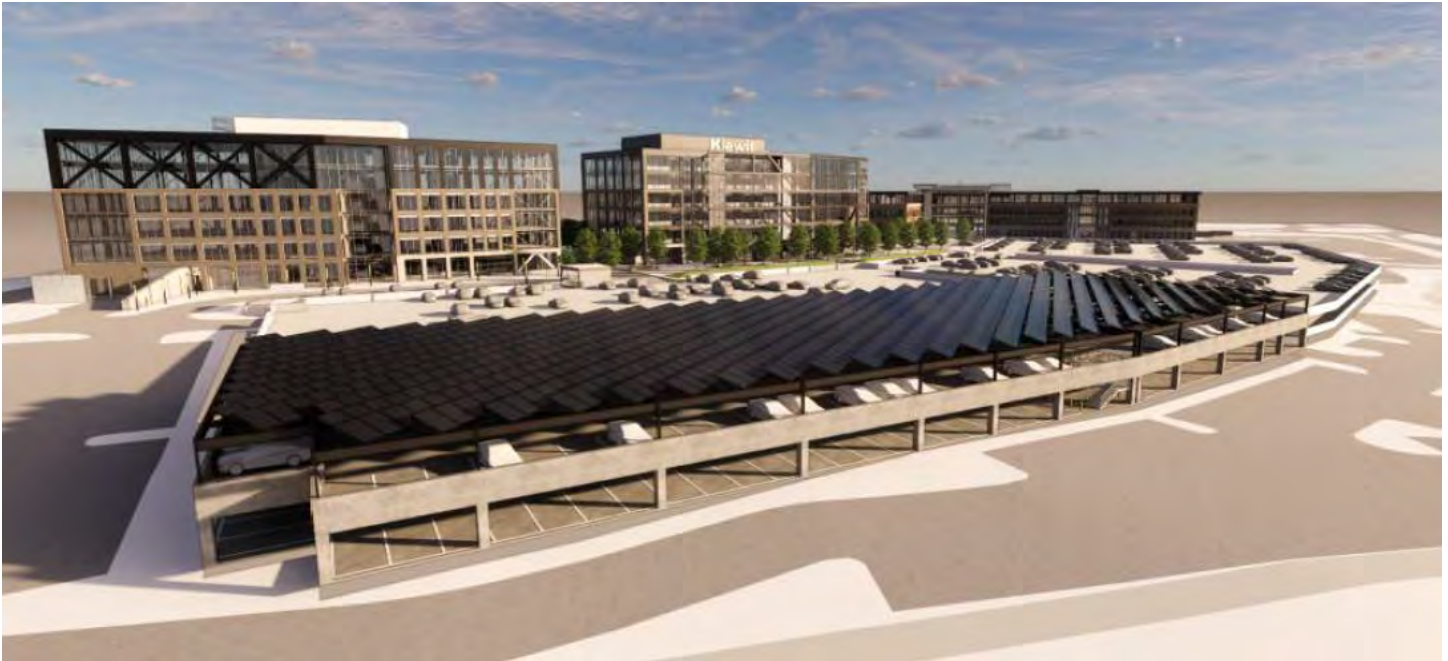
Exhibit 3: Solar Array on Parking Structure.
