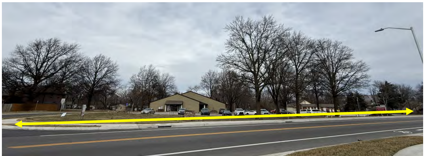
Exhibit 6: Sidewalk connection between the Green Prairie office building and adjacent church.
