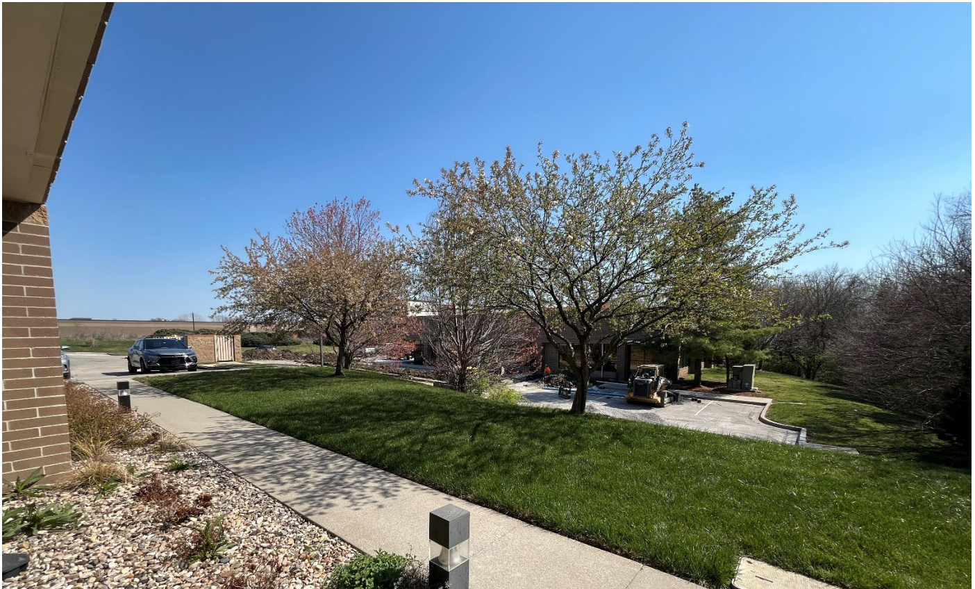
Exhibit 3: View of the north-facing facade of the Midwest Compounders building from the neighboring office building to the north.
