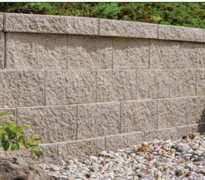
Wall Design Intent: Belgard Diamond Pro Meriam Blend Straight Face Retaining Wall or Approved Equal. Final block manufacture and color to be reviewed and approved at permit level.
