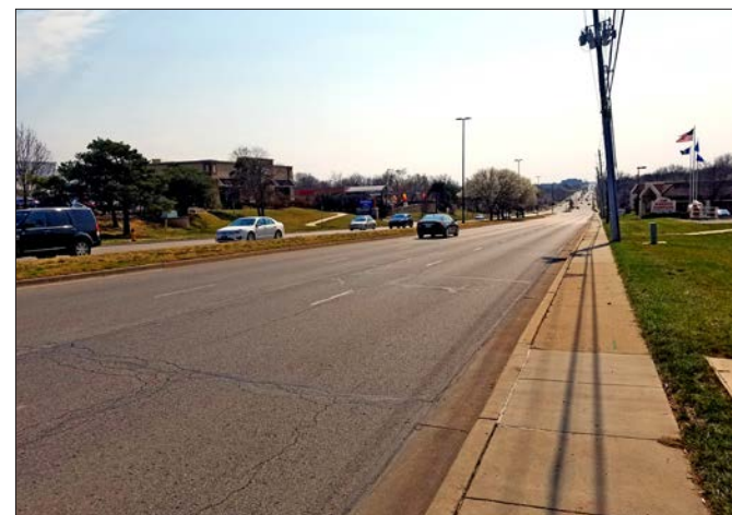
Existing sidewalks along Quivira Road between 97th & 99th Streets
