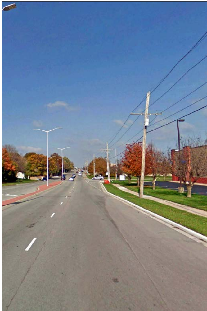
No pedestrian crossing opportunities exist between 95th Street & 91st Street
