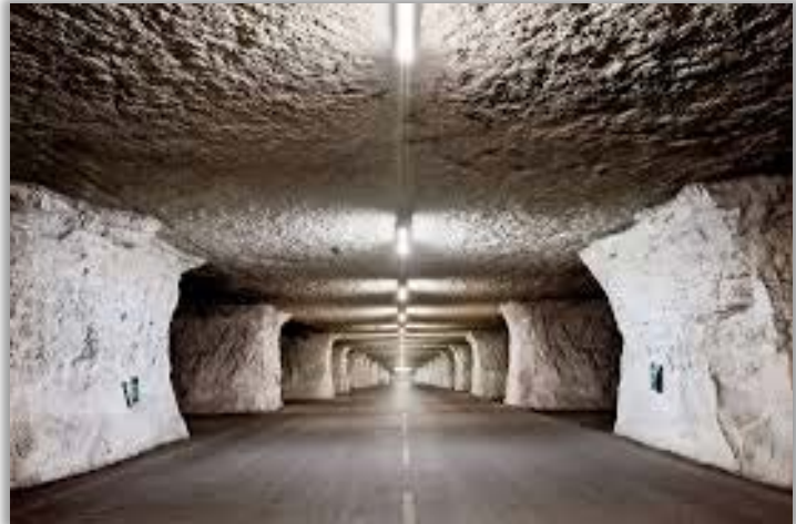
Meritex Underground Complex
