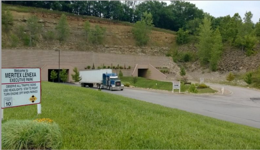
Main Portal into Meritex
