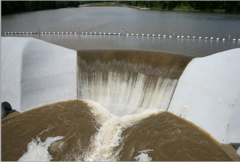
Water Dam at Lake Lenexa
